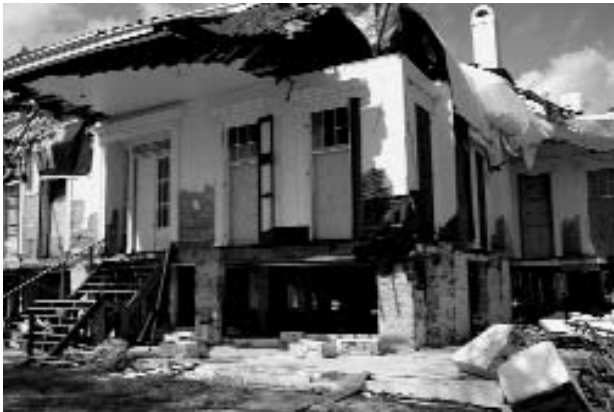
Beauvoir, Jefferson Davis' home, missing its wrap-around porch, Biloxi, Mississippi: 25 September 2005
