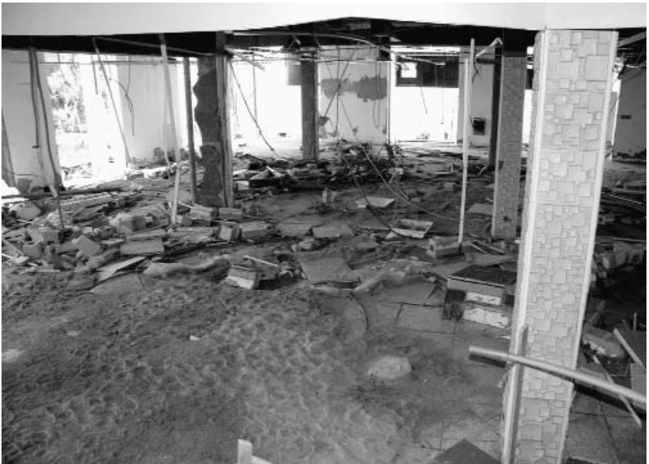
First floor interior, Gulfport-Harrison County Public Library, Gulfport Mississippi: 27 September 2005
