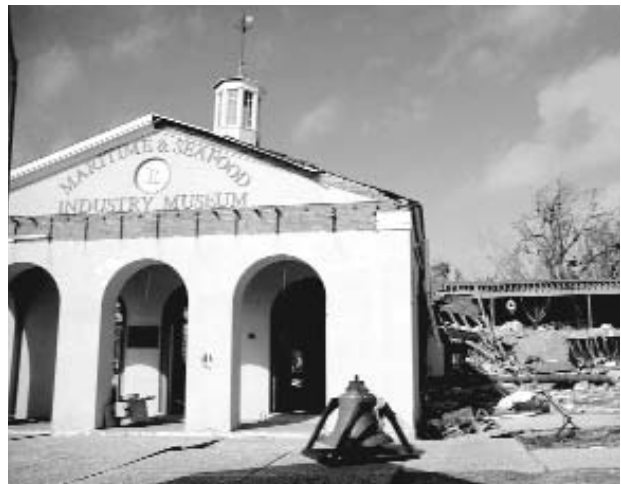
© AASLH Mississippi Team 1 Façade and building damage, Maritime and Seafood Industry Museum, Biloxi, Mississippi: 25 September 2005
