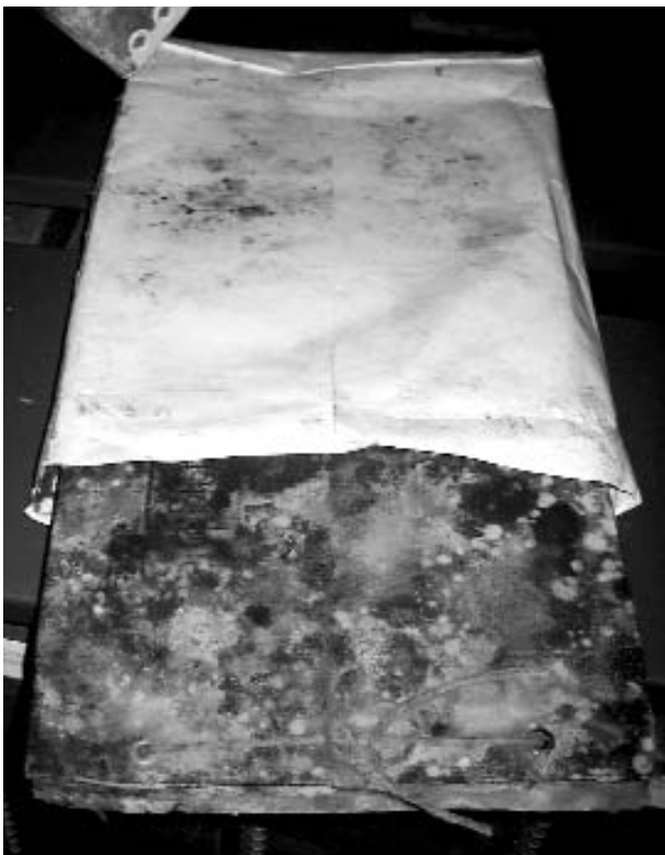
Tyvek envelope exacerbating mold damage, Biloxi Public Library, Biloxi, MS, 27 September 2005
