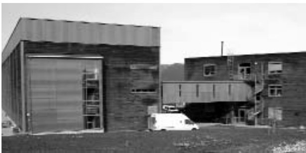
The automated storage
